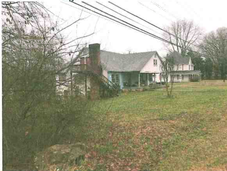
Neighborhood view south
