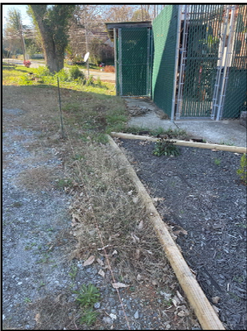
Above: Orange line denotes property line beyond fenced off area.
