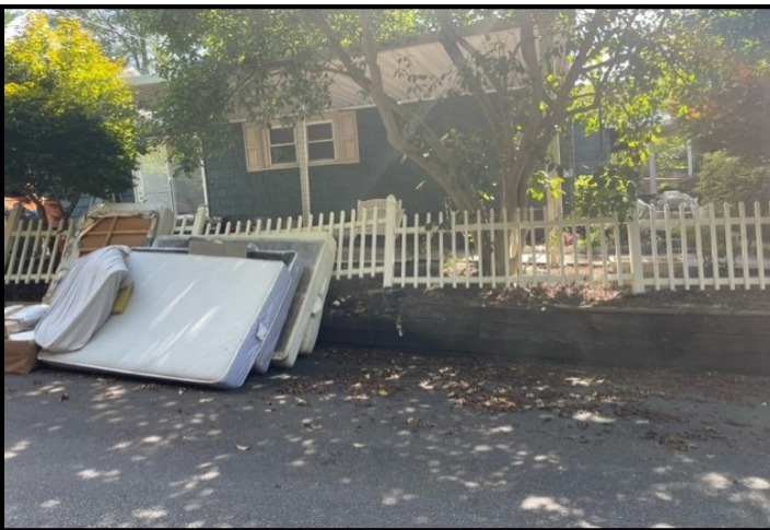
Above: Photos showing fence on west side of property.
