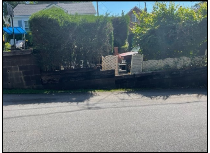
Above: Photo showing west side of property, concrete wall and fence
