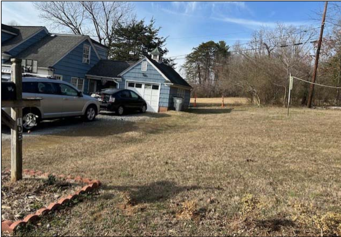
Above: House on site, pending removal
