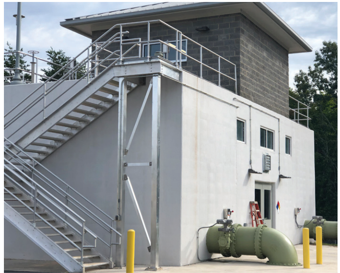
Lake Rhodiss WTP ActiFlo Building
