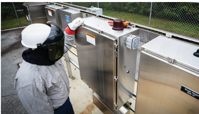
Example of proper PPE
