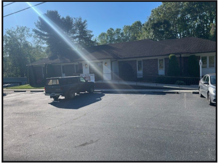
Front of site along Lower Creek Drive (sign behind truck indicating Farm Bureau is moving to Wilkesboro Blvd.)
