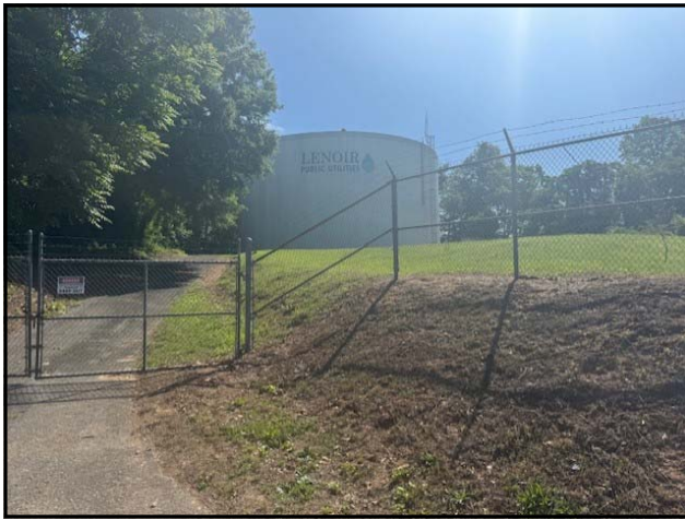
Above: View of water tower from Finley Avenue facing east.
