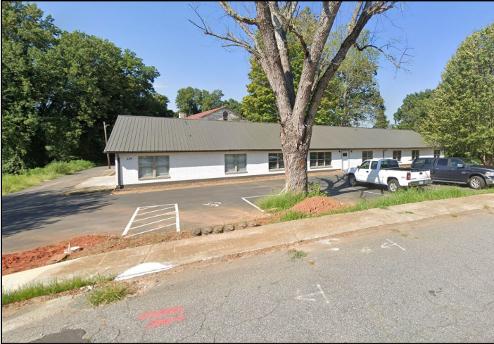
Below: Building 2, view from Wilson Street
