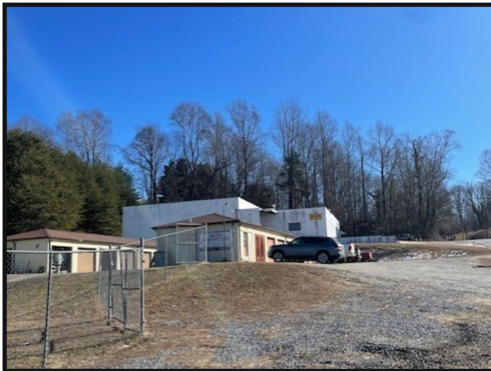
View of storage warehouse and chain-link fence enclosing porta-john and truck storage, looking south
