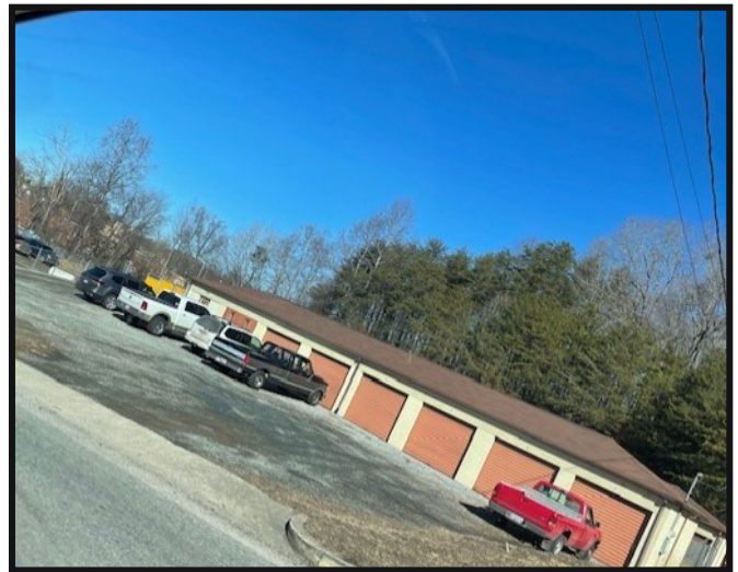
Mini-storage Warehouse on 729 Harrisburg property
