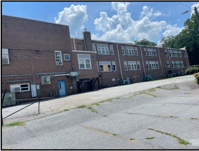
Above: Back of West Lenoir Elementary; auditorium (left), classrooms (right)
