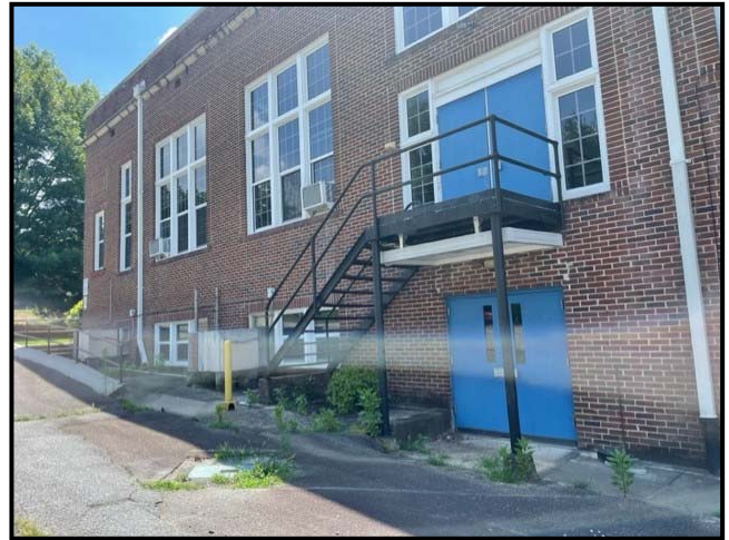
Above: Side entrance to Auditorium (top) and basement (bottom)
