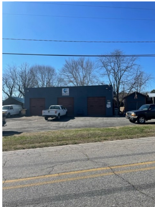
Walt Arney Wash and Polish building with three bay doors
