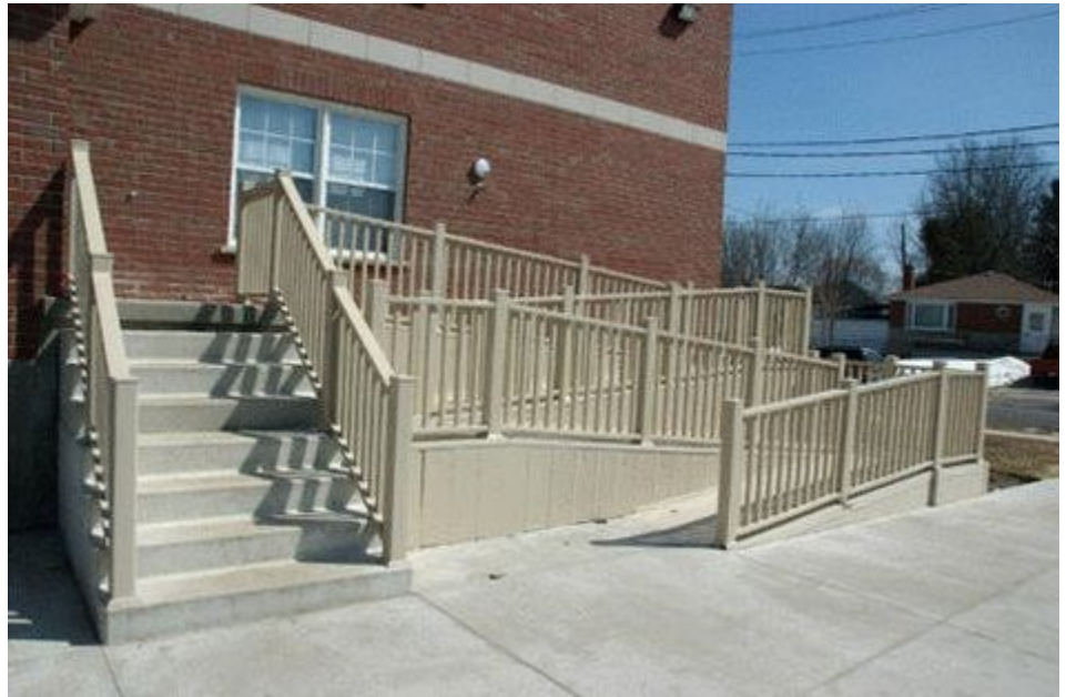
Photo shows an 8-step staircase to the left, and a switch-back ADA complaint ramp to the right.
