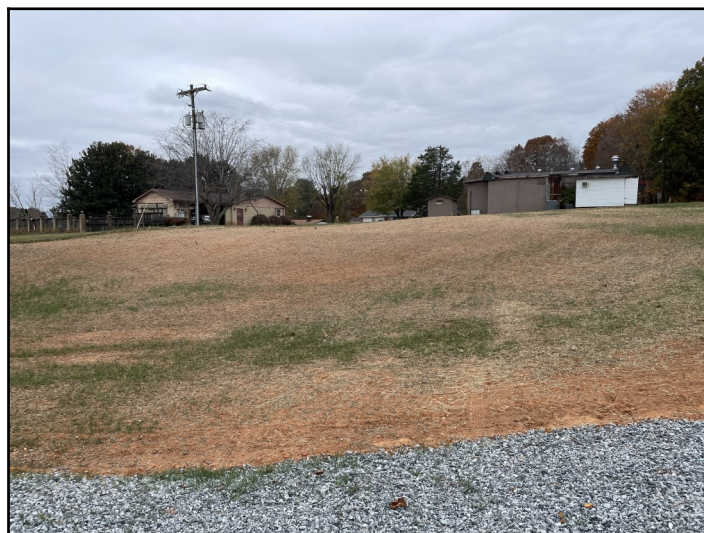
Above: Front of primary building facing Walt Arney Road
