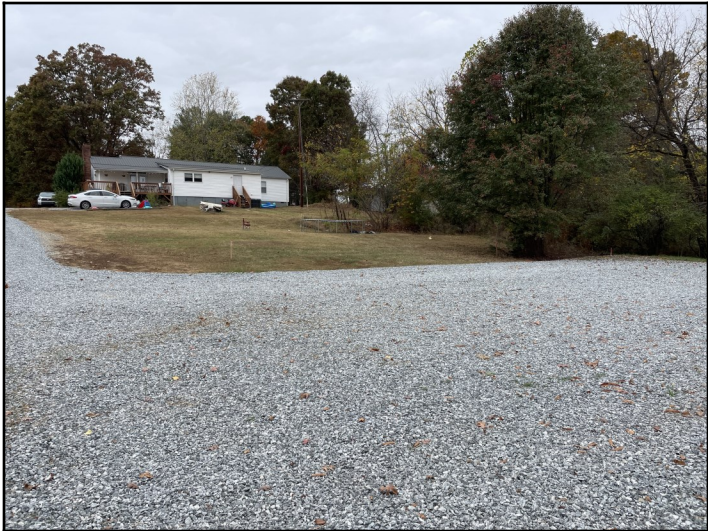
Below: Front of site identifying driveway and location of future landscaping buffer from residence
