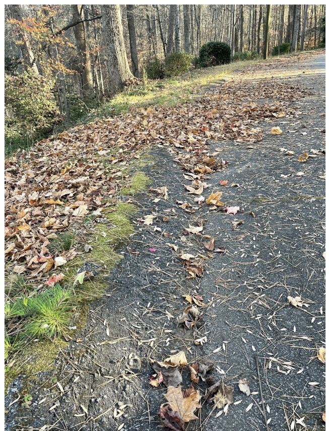
Below: Upper Hillhaven PI with valley curb
