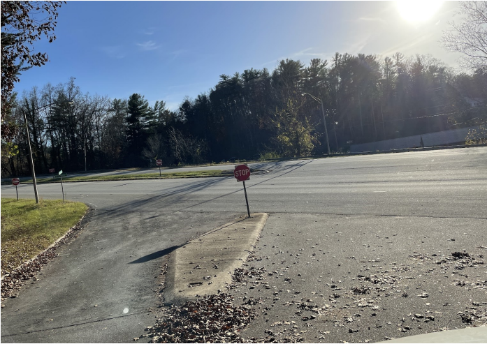
Above: Hillhaven Connection with US-321
