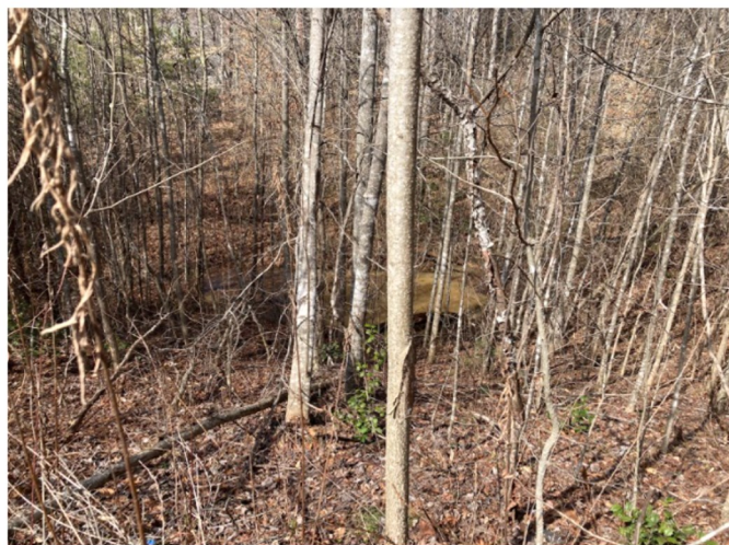
Basin holding stormwater following 1" rain event (Lot 16)
