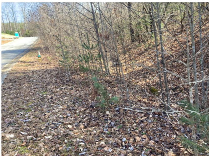
Stormwater conveyance swale on lots 6-8
