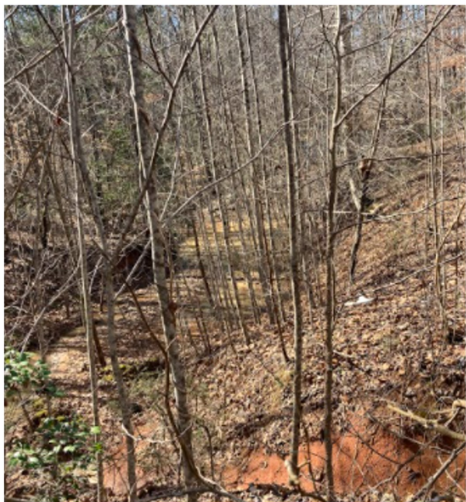
Erosion and channelization (foreground) on Lot 13; sediment basin holding water following 1" storm event (background).
