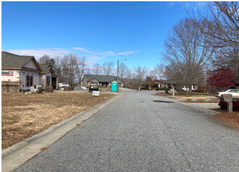
House under construction encroaches into the front setback.
