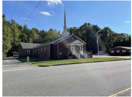
First Wesleyan Sanctuary facing Creekway
