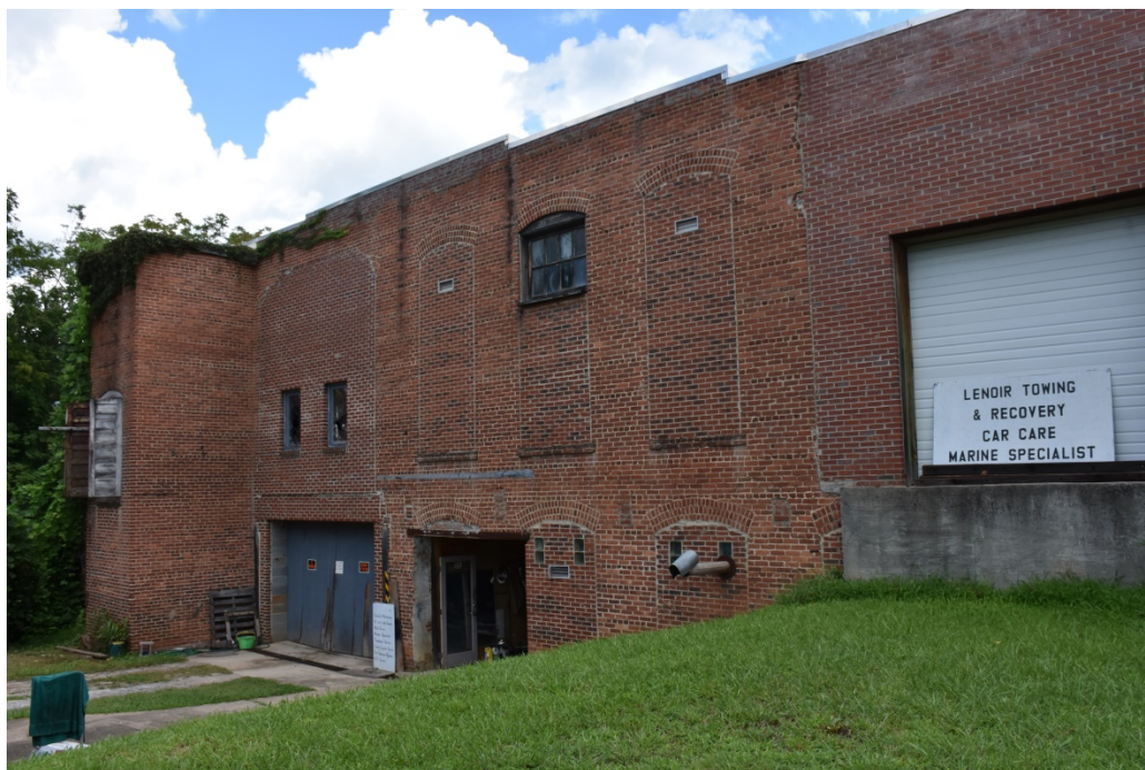
South elevation, looking northwest
