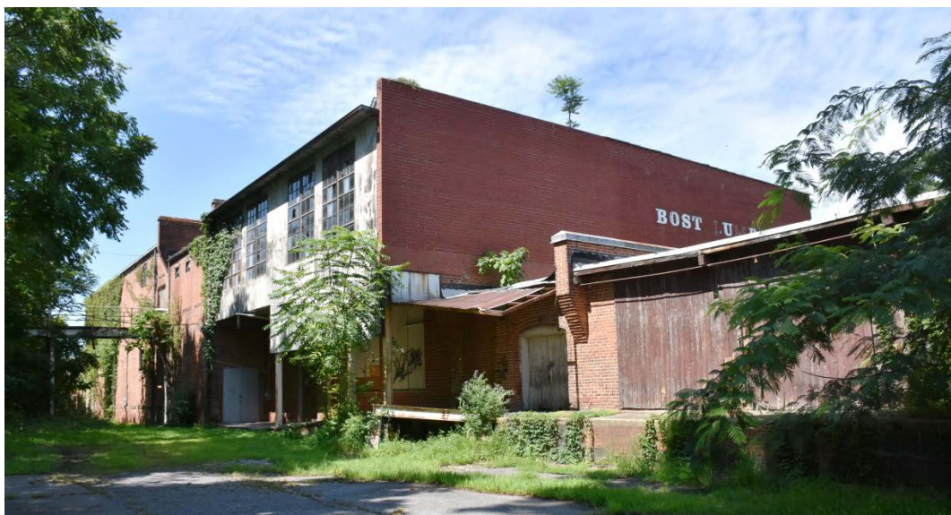
East elevation, north section, looking southwest
