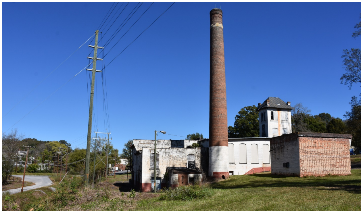
South elevation (above), October 26, 2018
