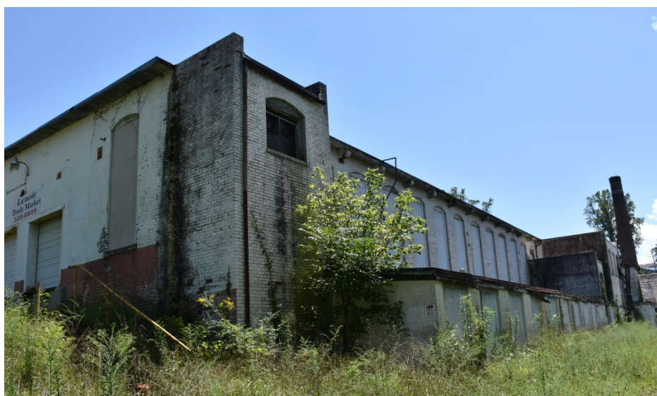
West elevation, north section, looking southeast
