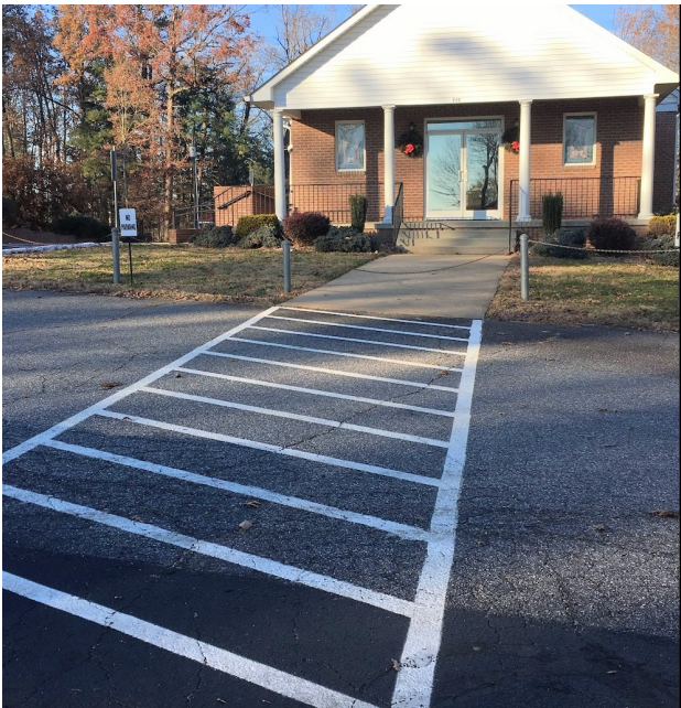
Above: Striped sidewalk across Stacey Place
