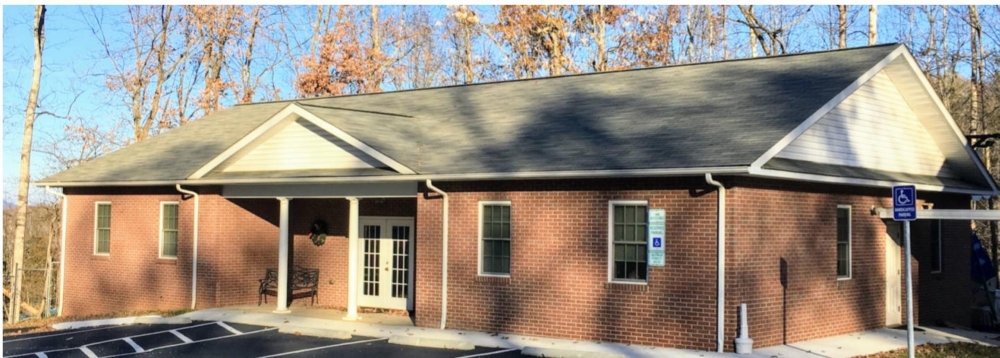
Above: View of church social hall from main parking lot
