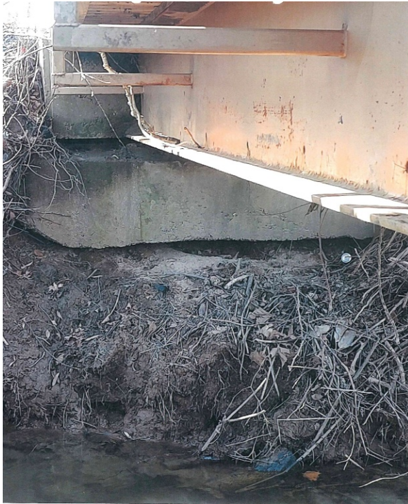
Figure 2 & 3: View at abutment requiring scour protection
