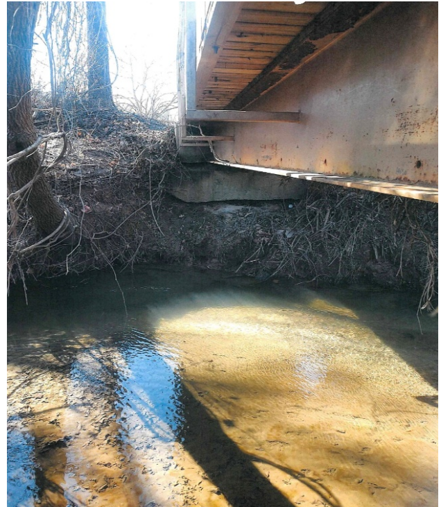
Figure 2 & 3: View at abutment requiring scour protection
