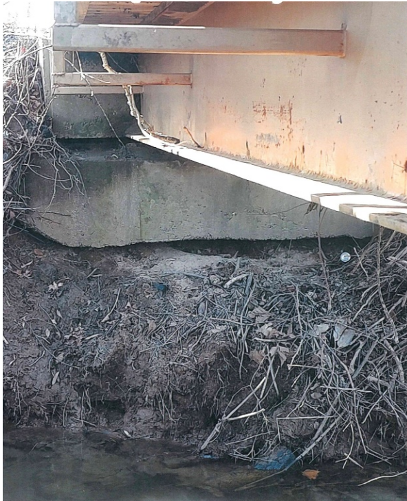
Figure 2 & 3: View at abutment requiring scour protection
