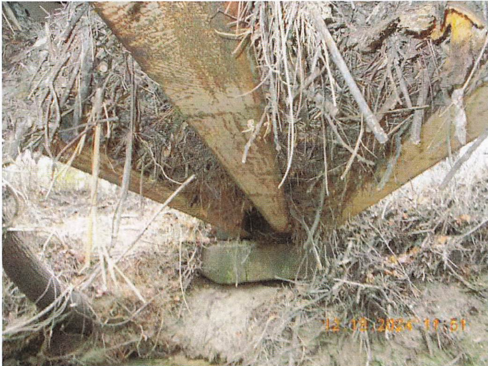
UNDERSIDE OF DECK
