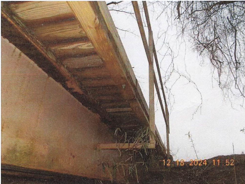
BRIDGE RAILING SUPPORTS
