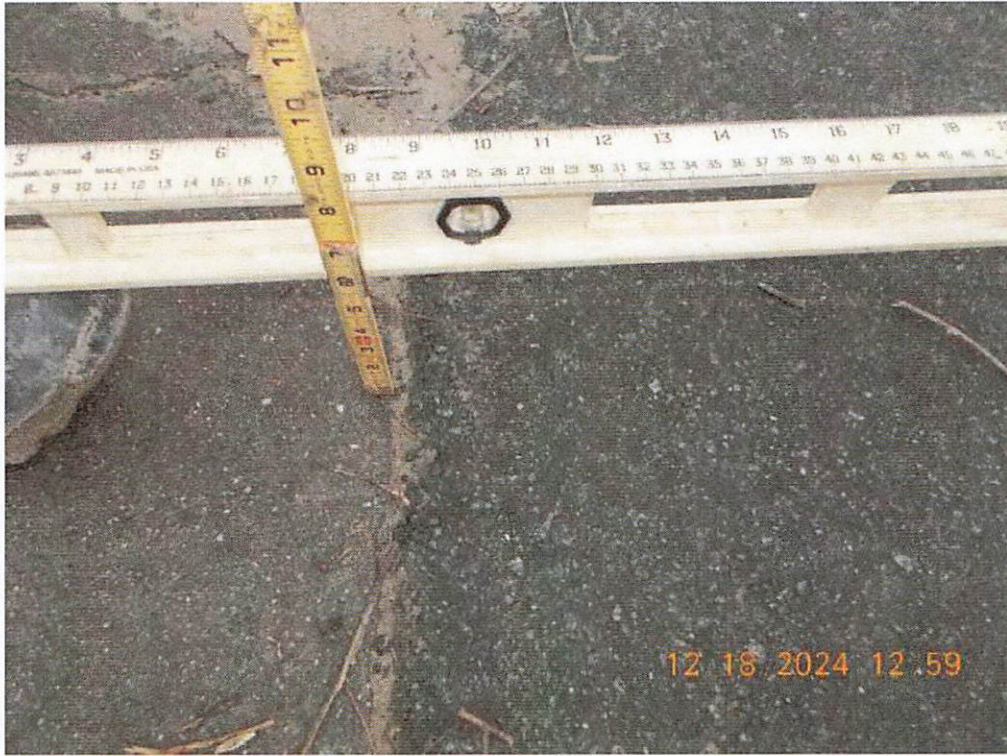
UP TO 6" OF SETTLEMENT IN WEST APPROACH AT ABUTMENT 1
