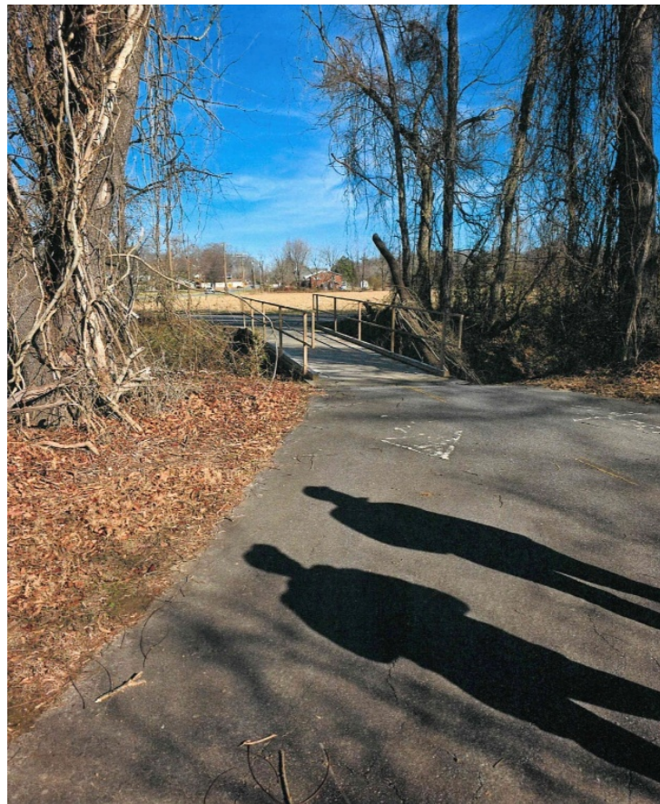
Figure 1: View at existing bridge
