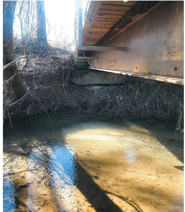
Figure 2 & 3: View at abutment requiring scour protection
