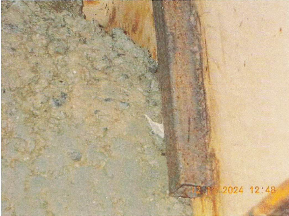
2" X 2" TUBING WELDED TO BEAMS AT ABUTMENT 1
