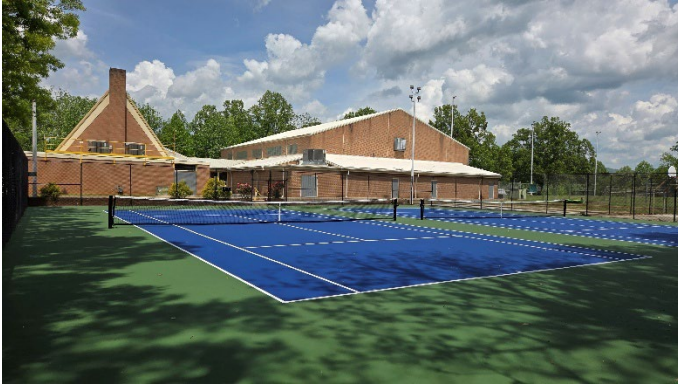
Tennis court resurfacing at MLK J. Center
