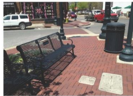
Red Clay Brick Pavers - Parkway
