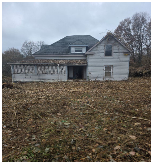
527 Prospect Street after abatement
