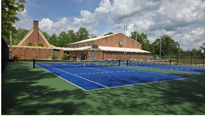
Tennis court resurfacing at MLK J. Center
