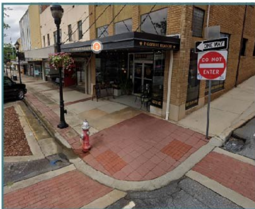
West Avenue and Church Street Intersection
