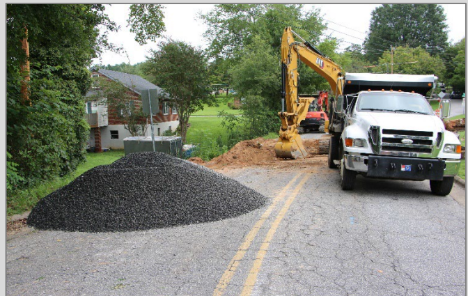
Powell Road storm drain repair
