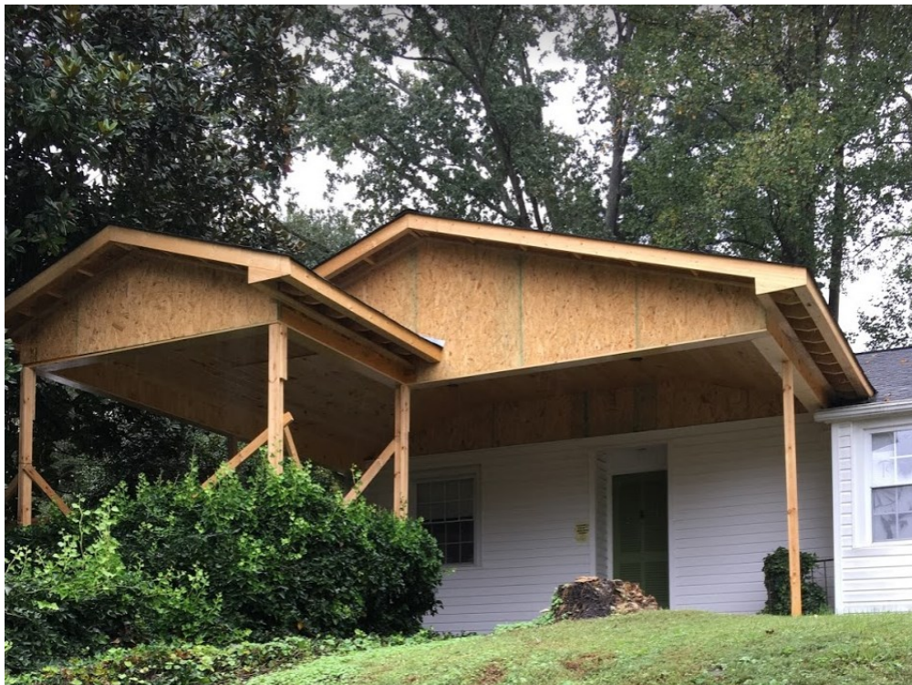
Project in progress
