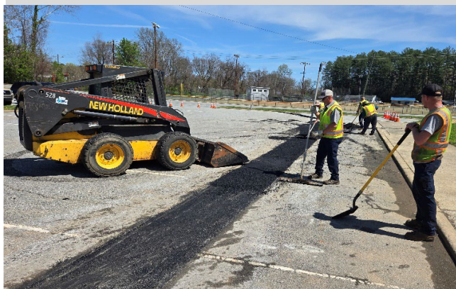
Street division patching storm drain cuts at Mulberry
