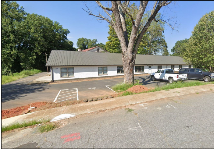
Below: Building 2, view from Wilson Street
