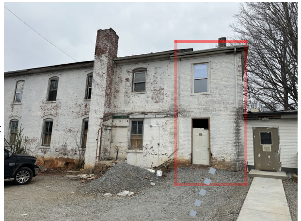
Above shows 10' wide area to be demolished to allow for building separation and new rear lot line.
