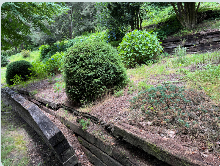
Existing Cross-tie Walls
