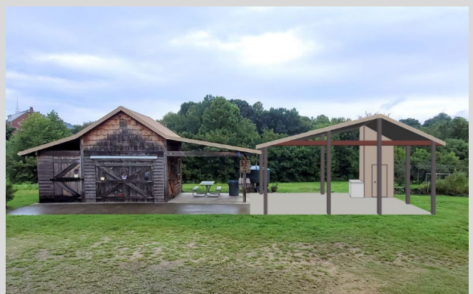
Teaching pavilion at Unity Park & Community Gardens
