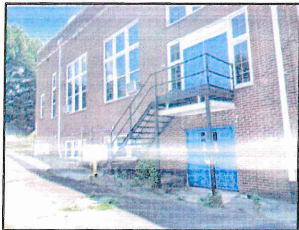
Above: Side entrance to Auditorium (top) and basement (bottom)
