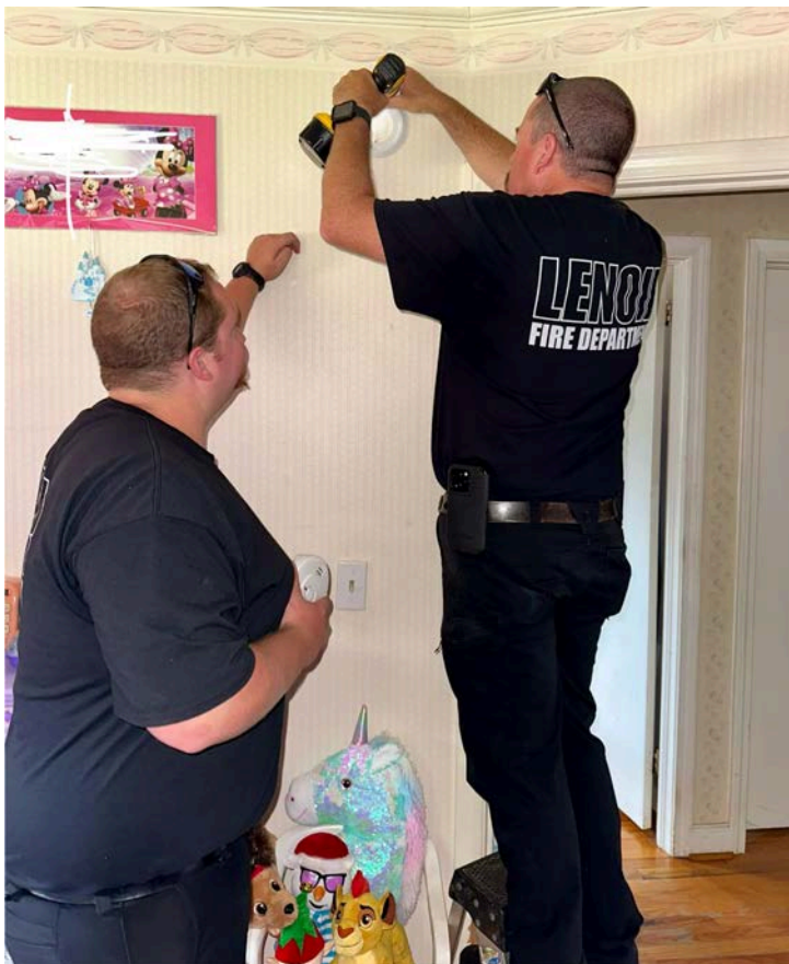
Staff installing smoke detectors during Smoke Detector Saturday.
