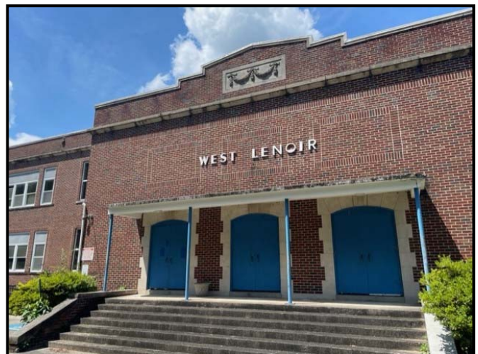
Above: Front of West Lenoir Elementary Auditorium where church service will take place
