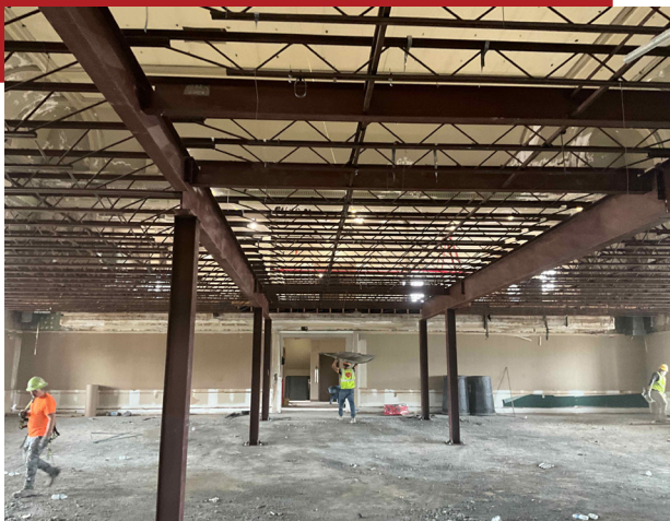
J.M. Cope carefully removed the structural steel piece by piece to reveal the original condition of the structure.
