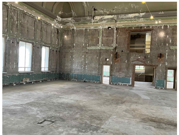
Completing this demolition during the design process revealed original historical elements that were covered up.
