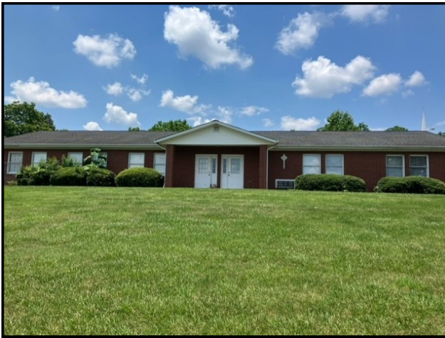
Above: View of Beall Hall (fellowship hall) from front of property
