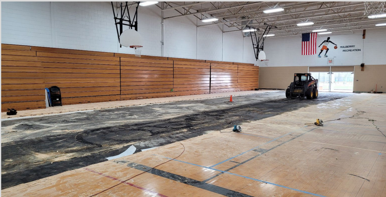
Mulberry Recreation Center Gym floor being removed
