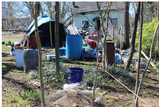
1216 Spainhour Street before abatement
