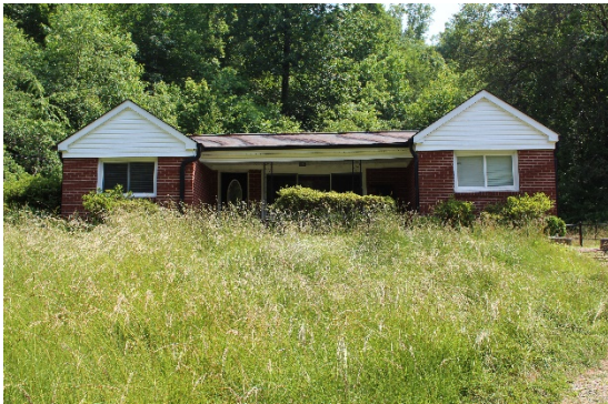
1415 Meadowlane Drive before abatement
