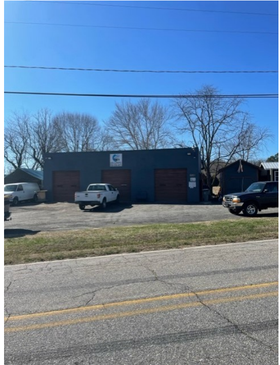
Walt Arney Wash and Polish building with three bay doors
