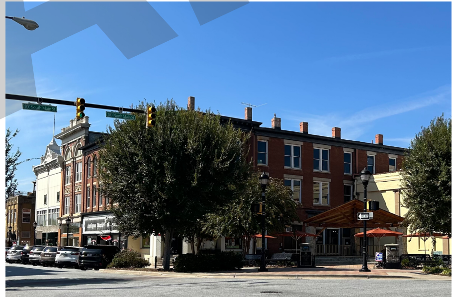
Northwest corner of West Avenue and Main Street, featuring the Downtown Stage and historic buildings. (October 9, 2022). DLR Group.
