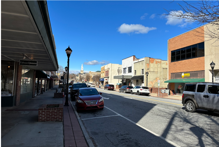
North Main Street looking north to the Caldwell County Courthouse. (January 23, 2023). DLR Group.
