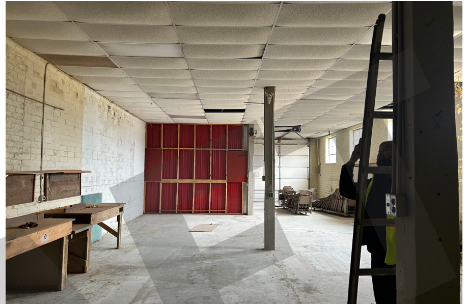
Interior of the Masonry Building. (December 15, 2022). DLR Group.
