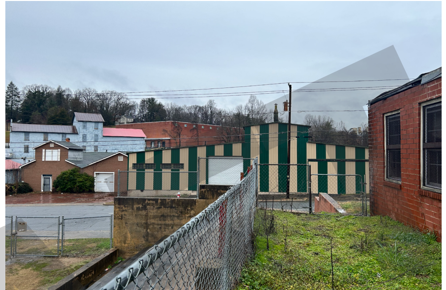
Future site of the OVT Pavilion/Farmers' Market, with the Masonry Building in the right foreground. (December 15, 2022). DLR Group.
