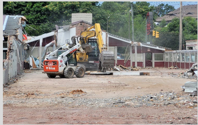
A.J.'s Steakhouse Demolition
