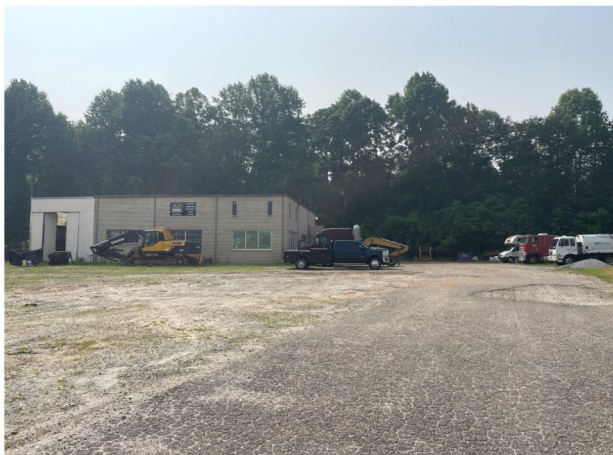
Existing building and customer equipment
