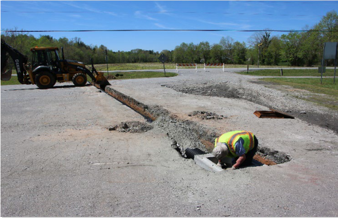
Drainage install at Powell Road parking lot
