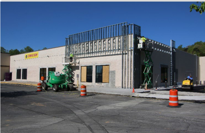
Planet Fitness construction
