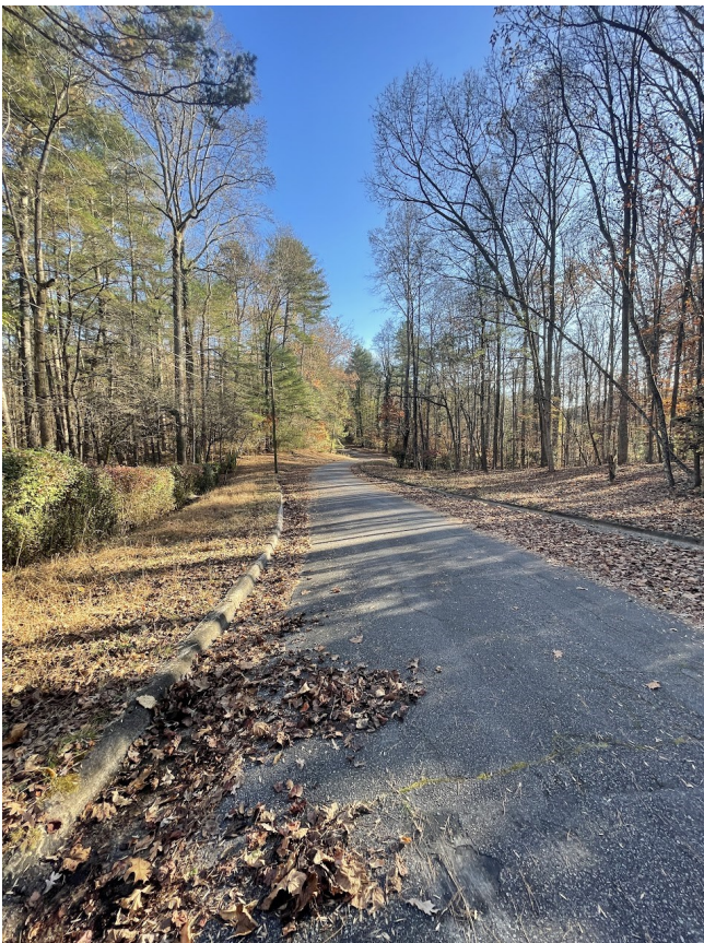
Below: Lower part of Hillhaven PI with curb and gutter shown
