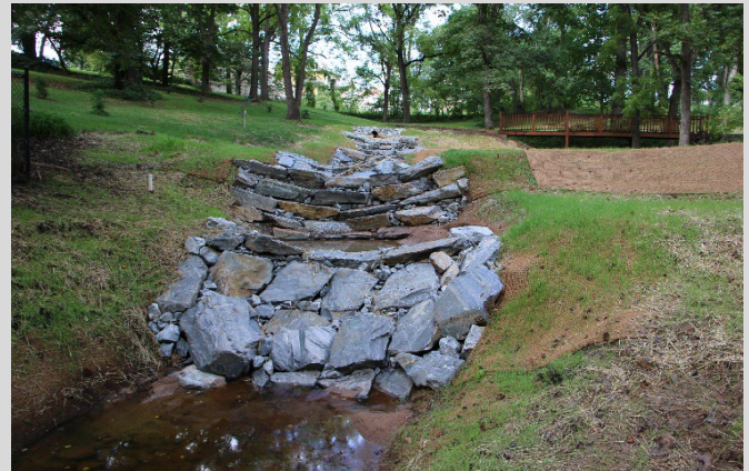
Stormwater feature at J.E. Broyhill Park
