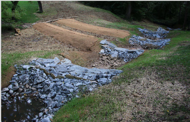
Stormwater feature at J.E. Broyhill Park
