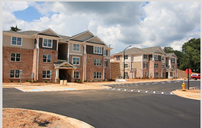
Kattz Coner construction
