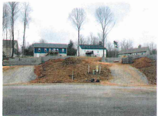
Homes under construction on lots 25-26 on Spring Time Court (foreground) and recently completed on lots 20-23 on Winter Place
