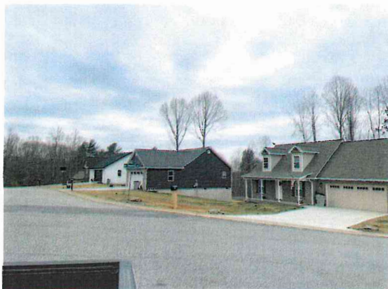
New Construction on Winter Place in Summerhill Phase I.
