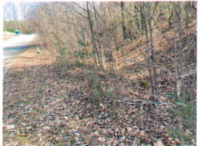
Stormwater conveyance swale on lots 6-8
