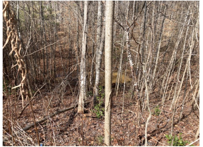
Basin holding stormwater following 1" rain event (Lot 16)
