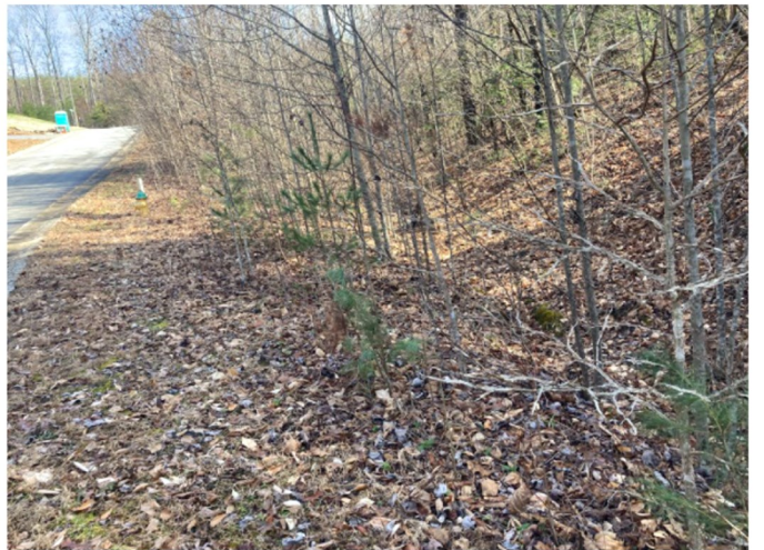
Stormwater conveyance swale on lots 6-8
