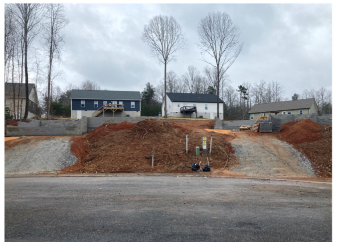
Homes under construction on lots 25-26 on Spring Time Court (foreground) and recently completed on lots 20-23 on Winter Place
