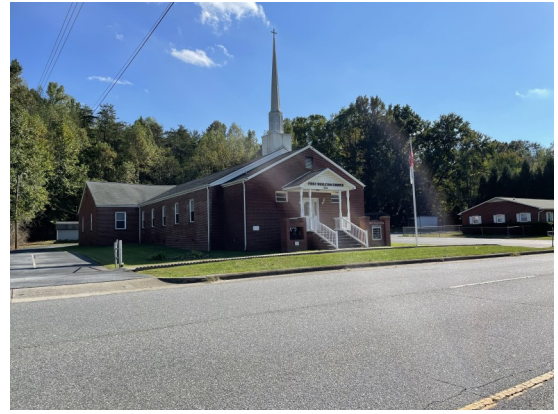
First Wesleyan Sanctuary facing Creekway
