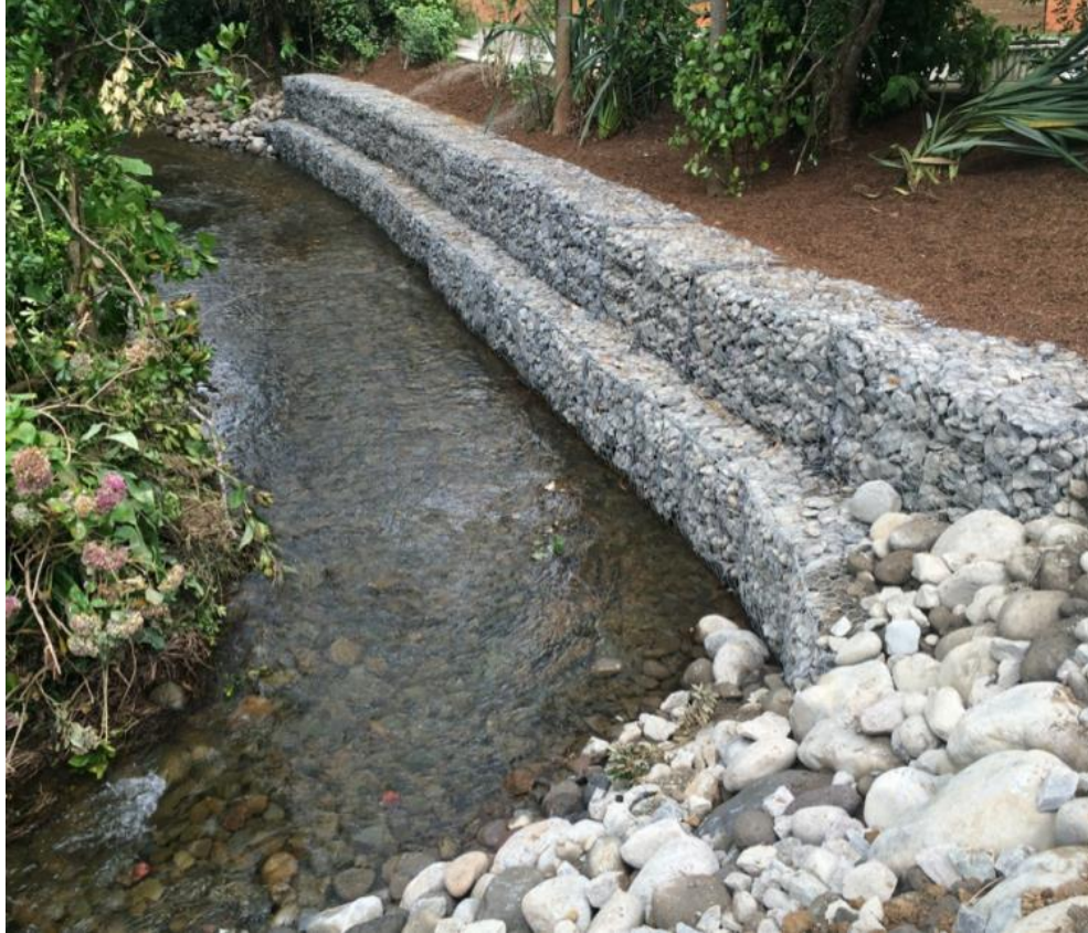
Gabion basket wall construction – Photo Credit- Warner Construction
