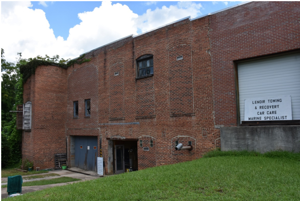
South elevation, looking northwest
