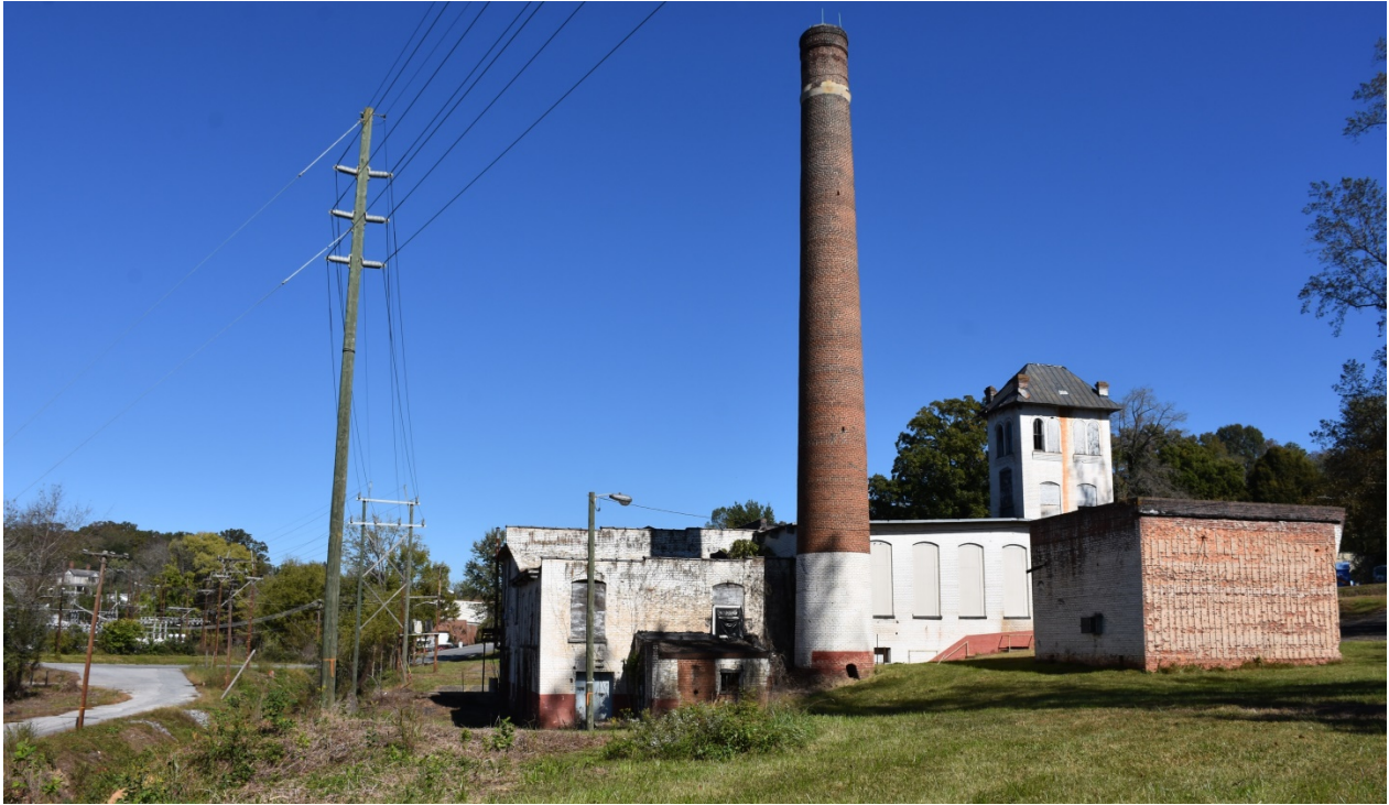
South elevation (above), October 26, 2018
