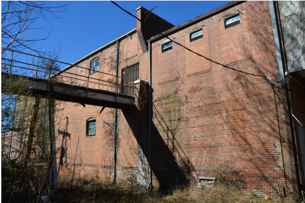
East elevation, south section, looking southwest
