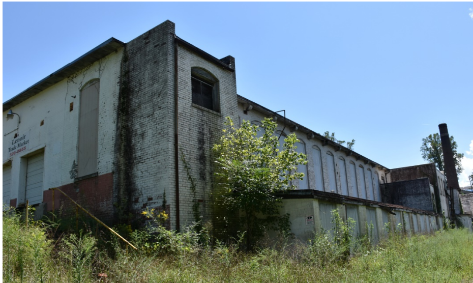
West elevation, north section, looking southeast
