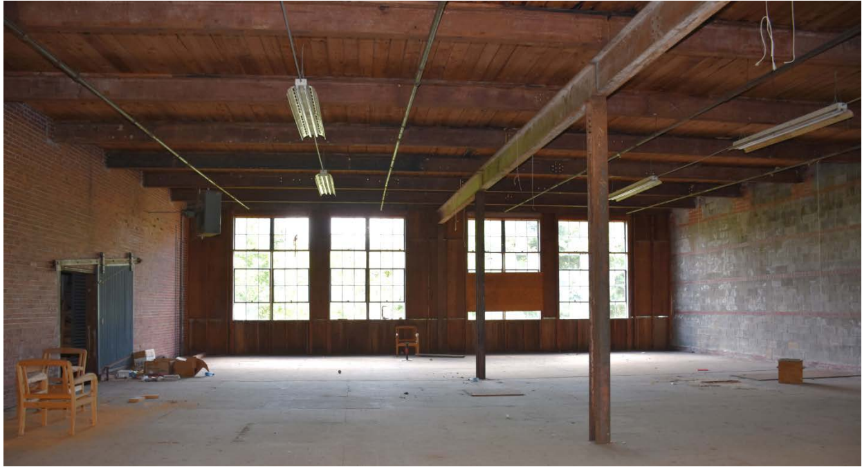
1950s addition, looking west
