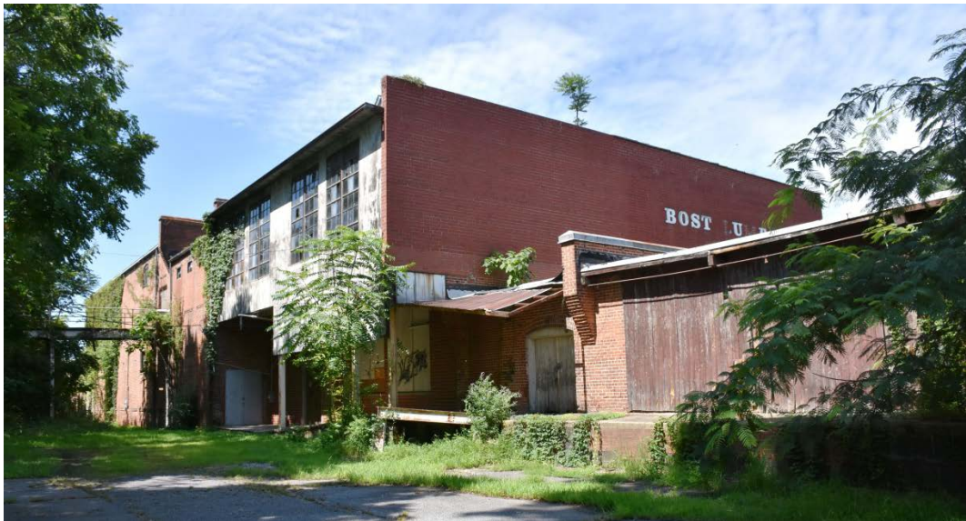
East elevation, north section, looking southwest
